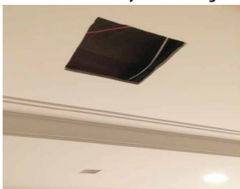
Cut Hole in Drywall Ceiling
